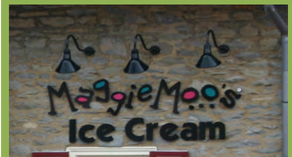
Externally illuminated sign, lit from above
